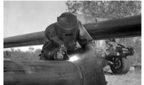
Fabricating a bend in a 12-in. gas line at the KMA Oil Field in Wichita Falls, Texas, in October 1938. The work was being done on a river crossing for the gathering system between some oil wells and the Phillips Petroleum Company cracking plant.
