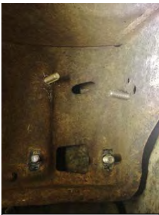
Opposite side, bolts installed
