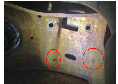
Holes marked, ready to go
